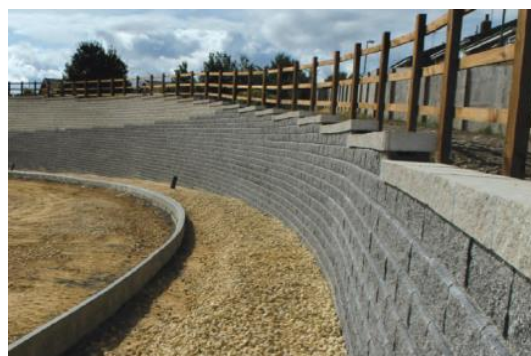
Figure: TensarTech TW System example.
