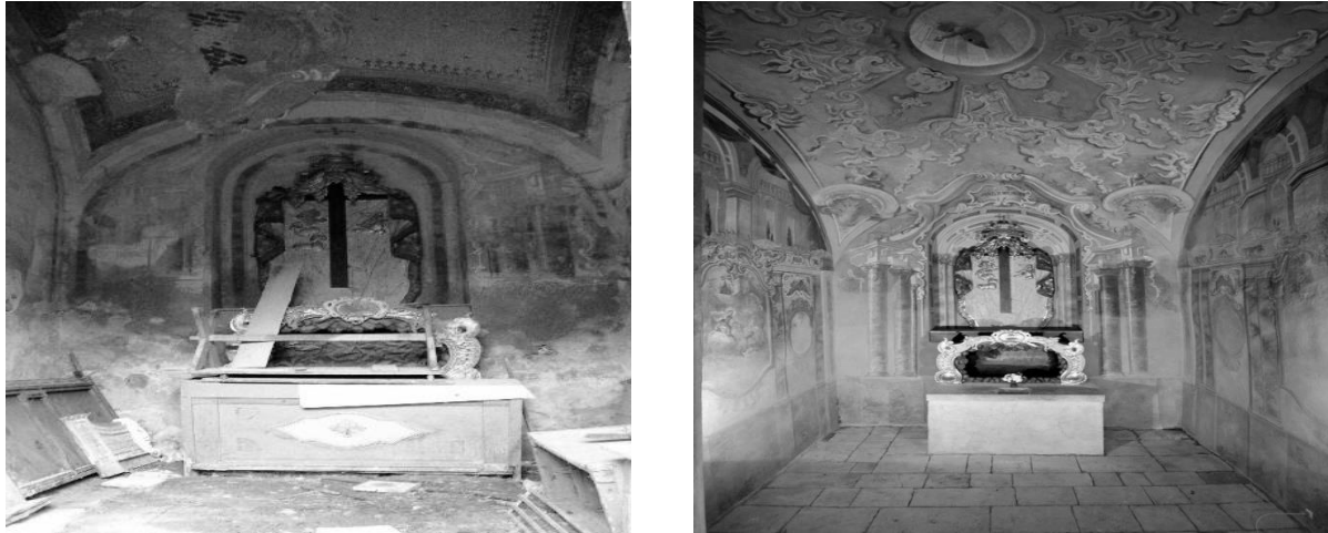
Fig. 6: Realised restoration works. State before and after the restoration.
