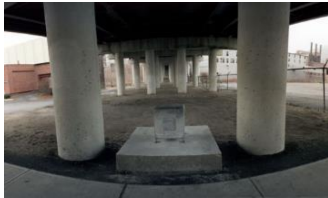
Figure 4: Harmonic Bridge , by O+A (Odland Bruce+Auinger Sam). An installation converts sounds from the traffic into music that is recorded through microphones and transferred to both sides of the road which it overlooks. Appeared in 1998 in North Adams, USA, http://www.massmoca.org/event_details.php?id=150
