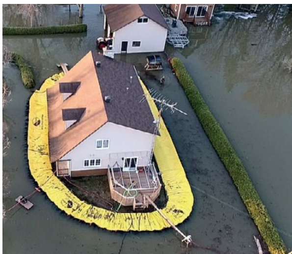
Picture 3: Building protection from flood waters Source:Quick Dam, 2020
