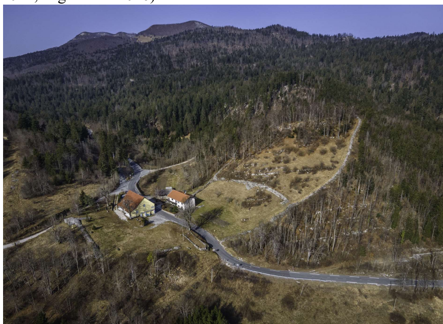
Fig. 2. Ad Pirum (Hrušica) from the south-east (photo S. Ciglenečki).
