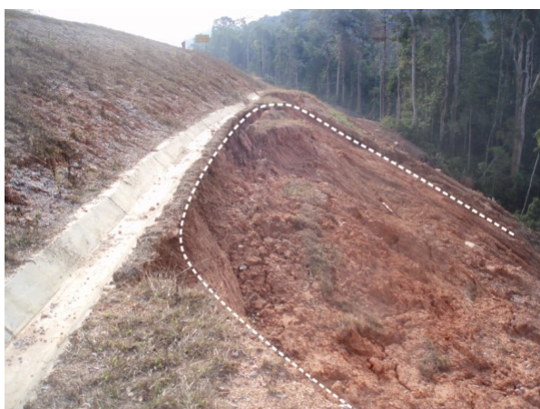
Figure 4: Drainage infrastructure (Hearn and Hunt, 2011)
