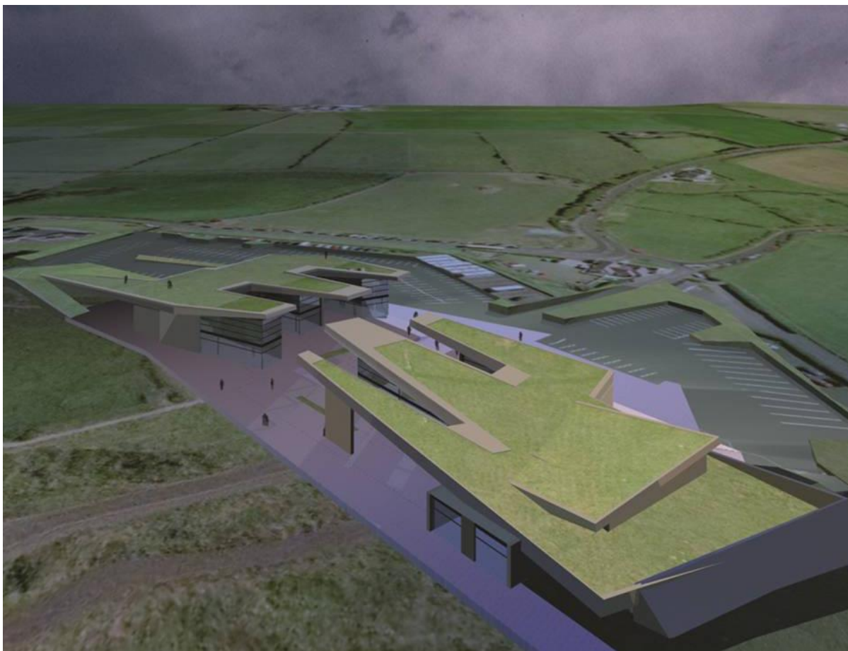
Img 13: Visitors' building for Giants' Causeway in Ireland; insisting on the concept of the continuity of the earth surface on the building structure. The roofs of the two separate building wings of the visitors' facilities complex were designed as planted surfaces, as parts of the surrounding landscape, as a continuity of the green surrounding terrain.
